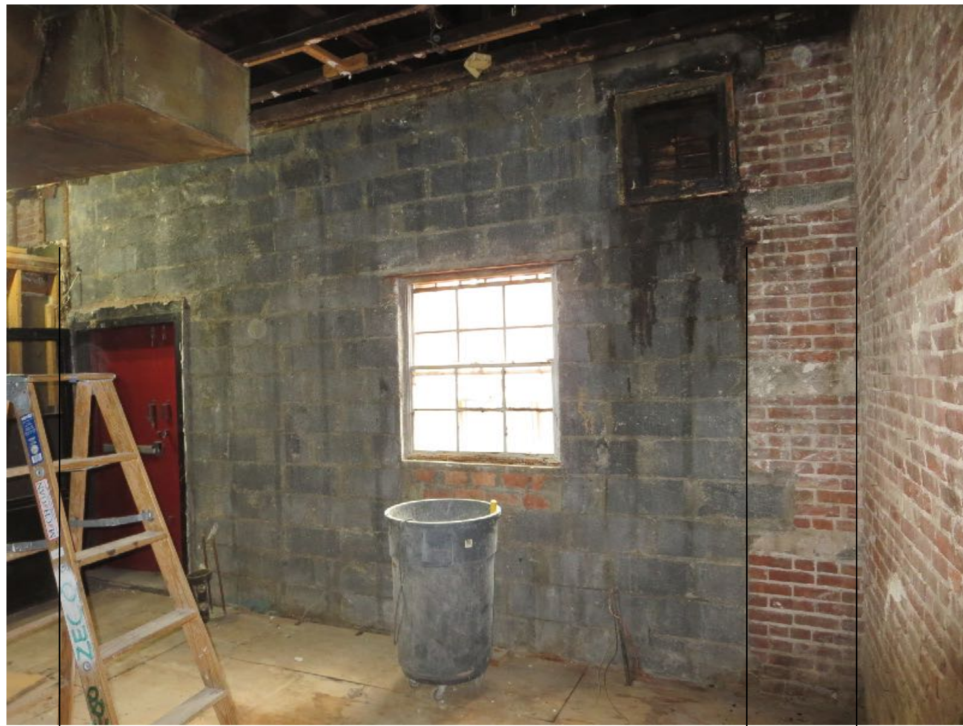
STOREFRONT C MASONRY PIER
