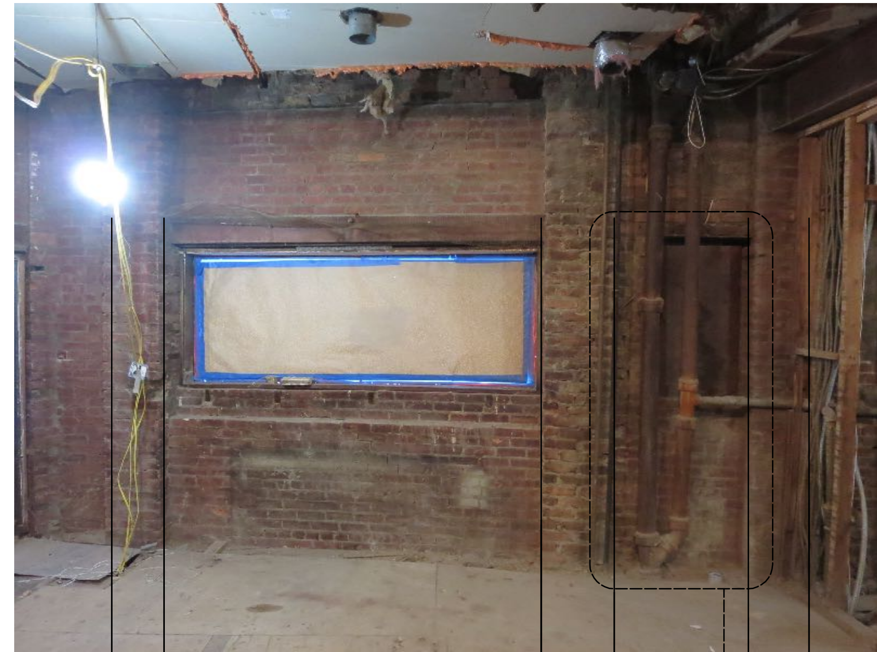
MASONRY PIER STOREFRONT B MASONRY PIER NEW DOOR IN HIST. LOC. MASONRY PIER
