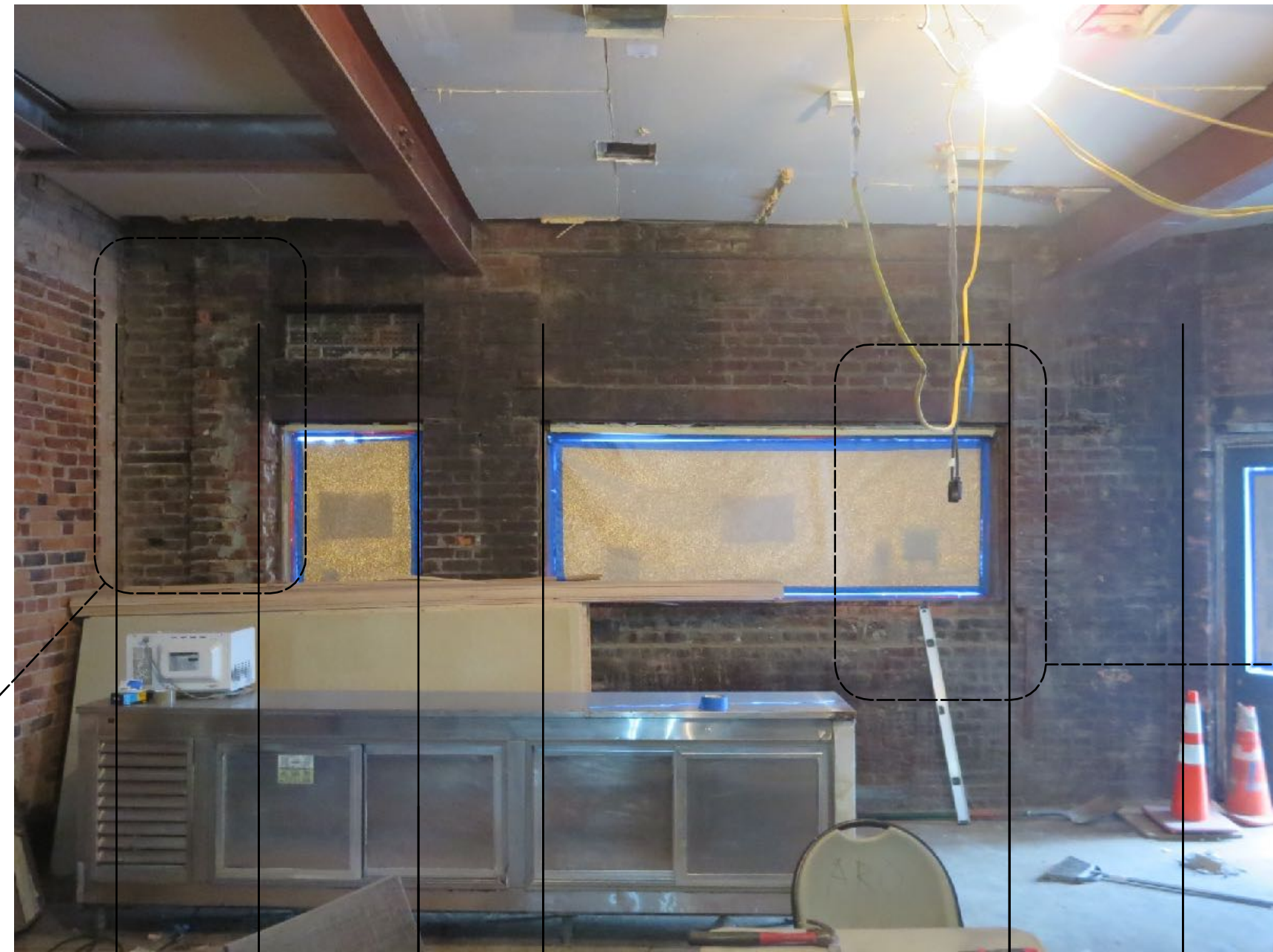
STOREFRONT "A" FAILING COLUMN
